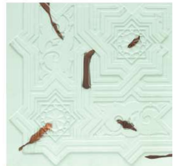
VC03 - Damaged Tin
